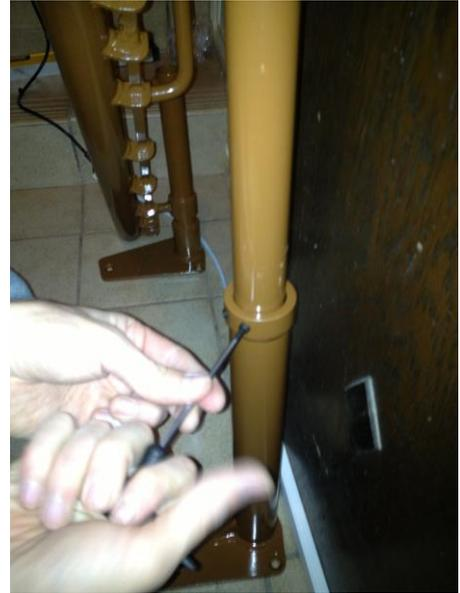
**Step 6:** When all rail parts are connected and all pillars are set to the correct height check again all clearance measures and the correct position of the rail according to the installation drawing.
