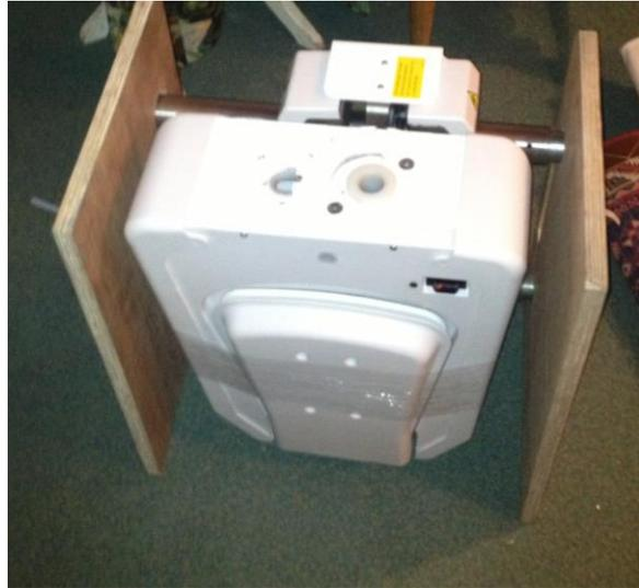
**Step 2:** Take off the wooden plates on each side. Put the drive unit on the floor (use protection under it so not to scratch it). Then 2 people should lift the drive unit on the rails and attach the installation rails to the top of the installed rail on the staircase. Then slide the drive unit down until it reaches the top of the installed rail. Use the handwheel to drive the unit onto the installed rail so that the lower rail passes entirely through the lower trolley.
